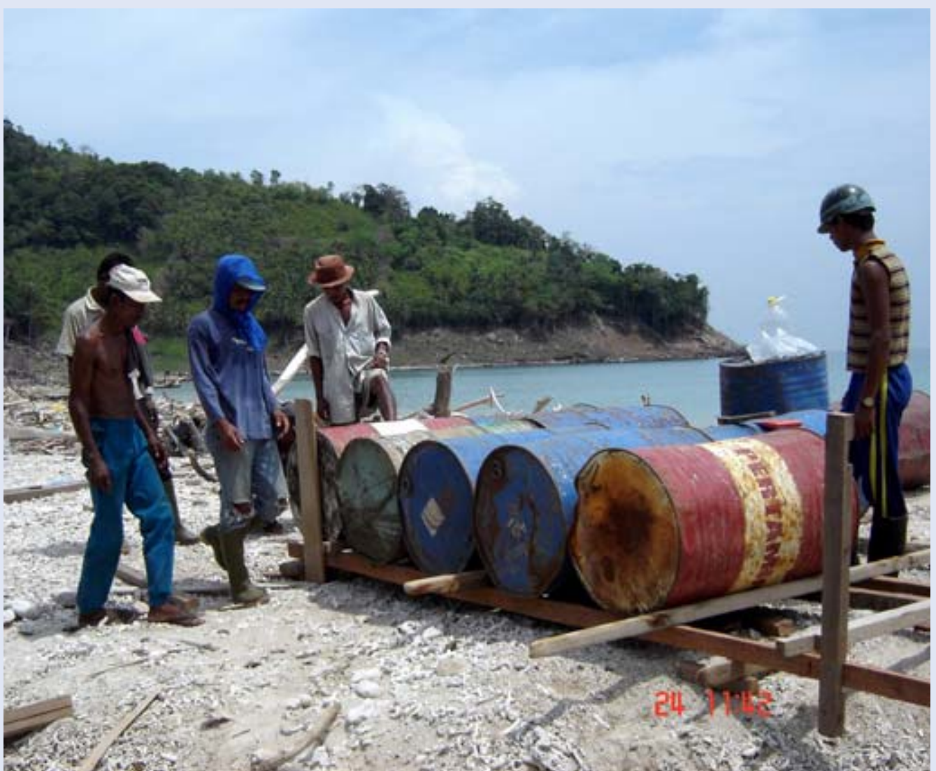
Pulo Aceh people making floating pier in Luen Bale..
